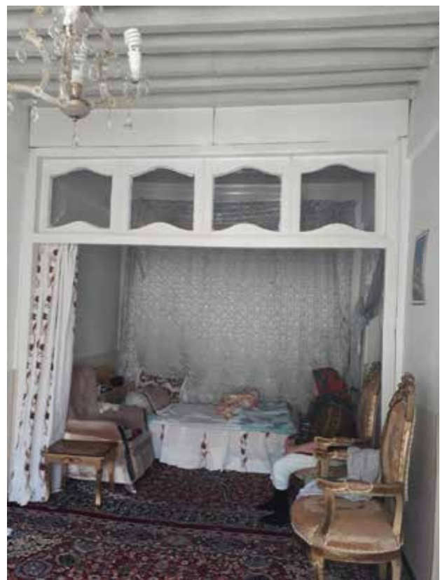
Fig. 5. Two wooden separators in houses 2 and 4. Source: authors' archive.
