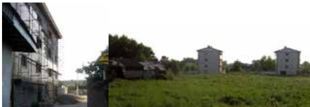
Fig. 3. Building on agricultural land, regardless of surrounding texture (right) and extensive construction in narrow alleys (left). Source: authors' archive.
