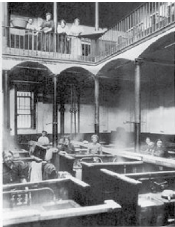
Fig. 1. Public Bath of Fredrik Street in Liverpool, UK. Source: bkthisandthat.org.uk.
