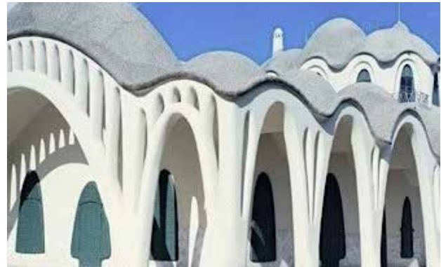
C) Nature-inspired Branches in the Structure of Columns, Masia Freixa. Source: www.catalunya.com
