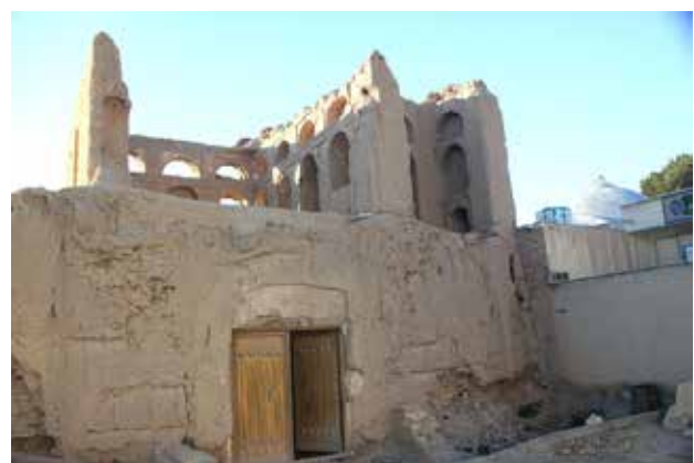
Fig. 3. Eastern View of Bani Ameri House from Outside. Source: Authors' archive.
