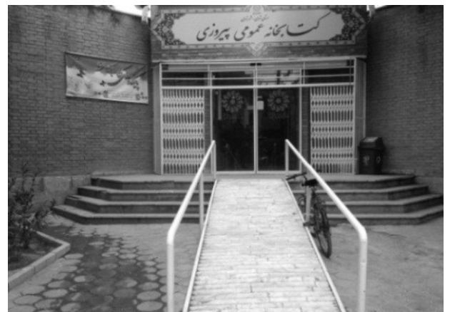
Fig.6. Inaccessibility of Public buildings. Piroozi Park (district 13) Photo: Neda Rafizadeh, 2016.
