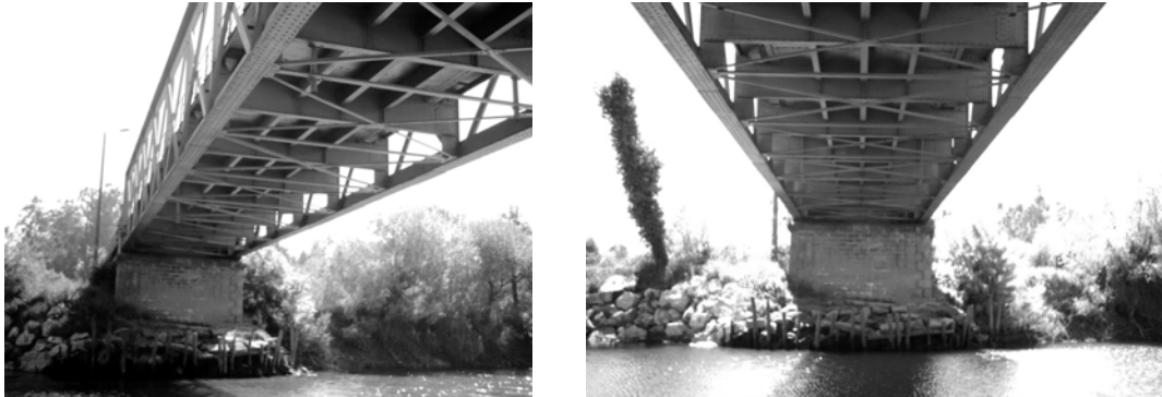
Figure 4. Bottom views of the S. João de Loure bridge: bracing system (Furtado et al., 2003)
