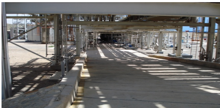
Figure 1. A view of pipe supporting structure
