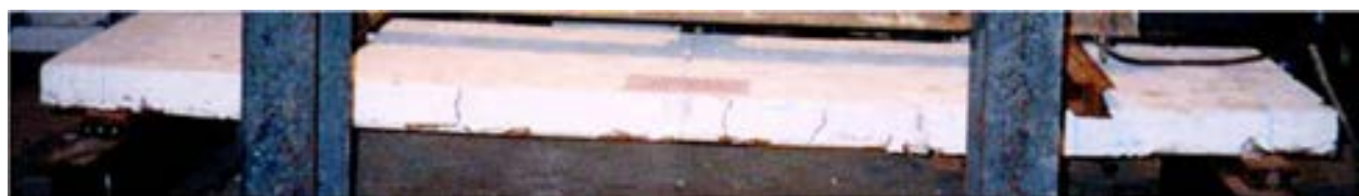
Figure 13 Crack formation for 525- to 675-mm shear span at the ultimate stage.
