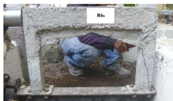
Figure 11 Central top bracing frame filled with concrete.
