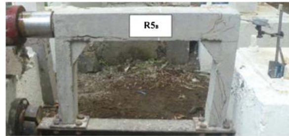
Figure 10 Corner top bracing frame filled with concrete.
