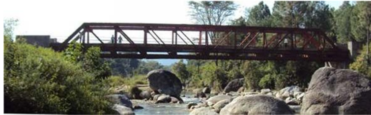
Figure 1 Side view of 40-m steel truss bridge.
