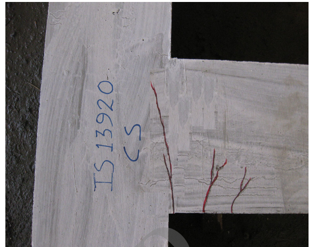
Fig. 11 Crack pattern of IS 13920 CS
