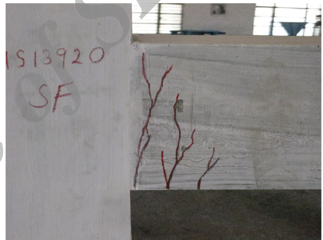
Fig. 12 Crack pattern of IS 13920 with SF
