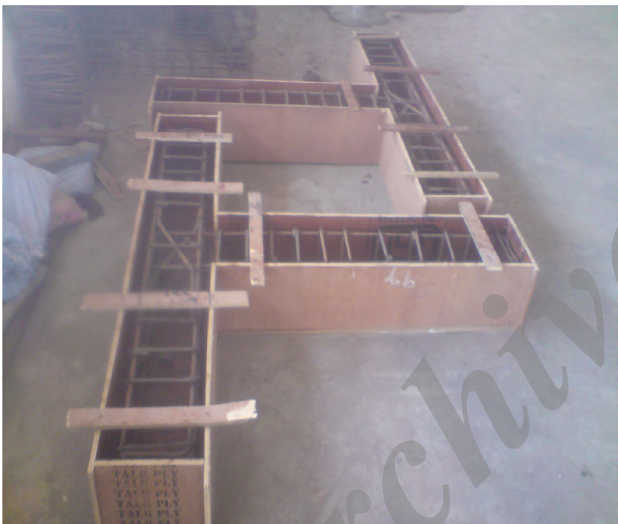
Fig. 3 Formwork and reinforcement
