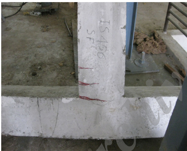
Fig. 10 Crack pattern of IS 456 with SF
