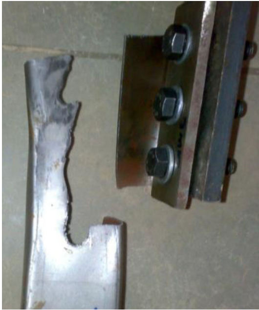
Fig. 41 Block shear failure of 1.5 mm thick sample specimen using 5 mm thick packing plate
