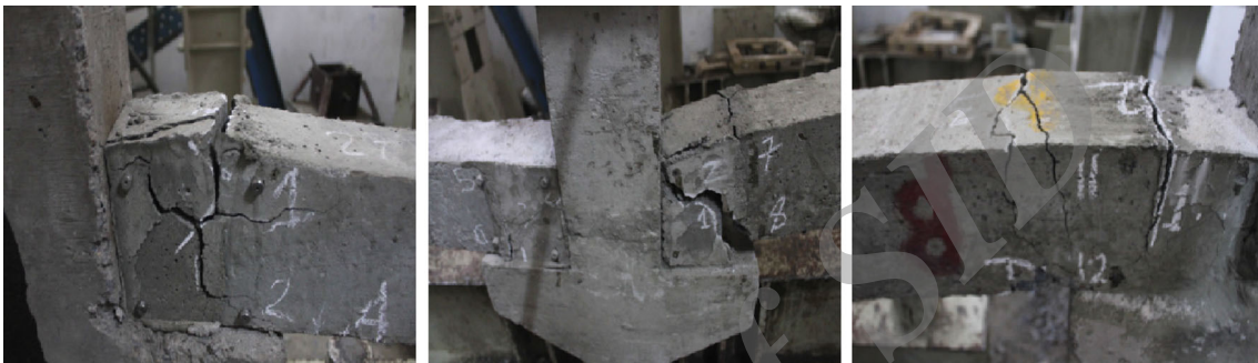
Fig. 12 Crack formation in specimen PC-CRW
