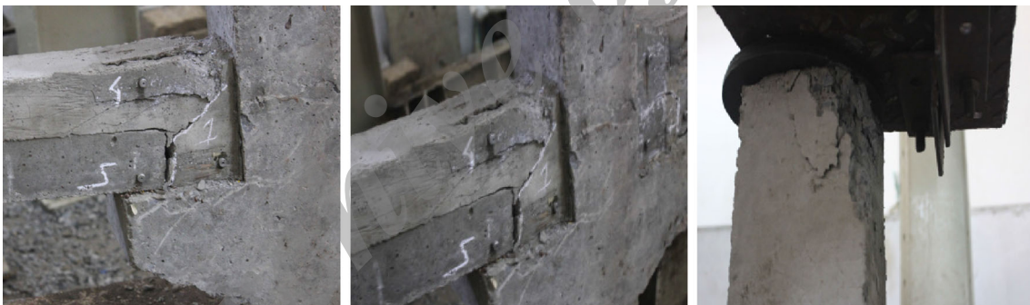
Fig. 13 Crack formation in specimen PC-CRS
