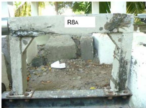
Figure 8 Epoxy repaired, with partial concrete infill corner-braced frame.
