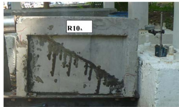
Figure 10 Epoxy repaired, with concrete infill diagonal-braced frame.
