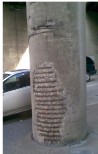
Fig. 2 Bridge column, Howe Ave., Akron, OH, USA
