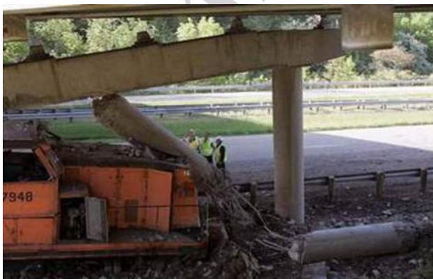
Fig. 1 Detached cap from girders due to a railroad locomotive collision on I-74 at I-275 intersection in Cincinnati, OH
