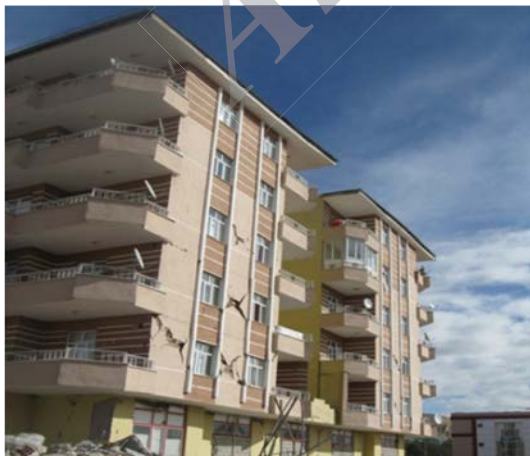
Fig. 1 A view of the prototype building
