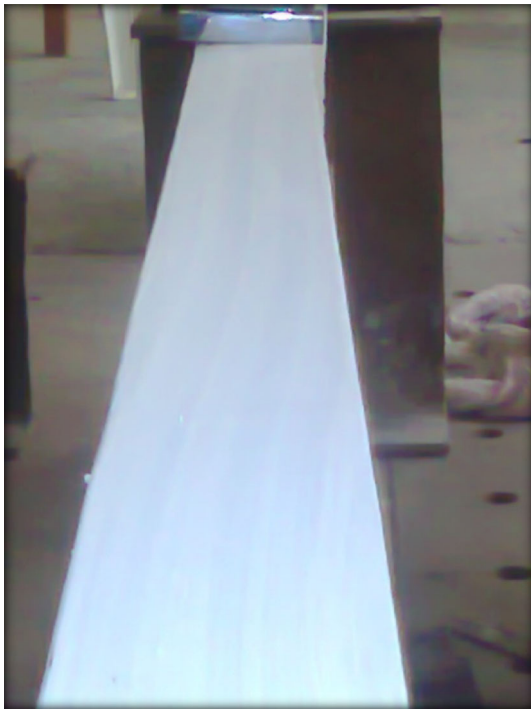
Fig. 16 Lateral movement of beam SBWO5 (lateral torsional buckling)
