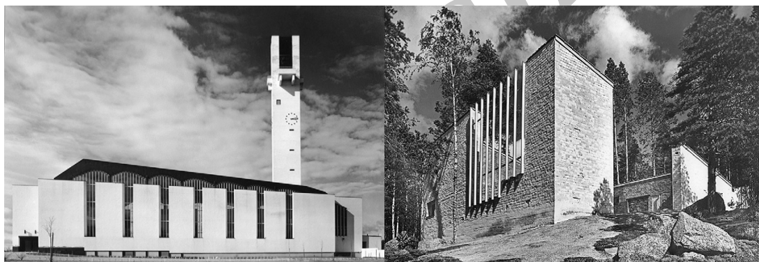
▲ Figure 1. Church of the Plains by Aalto, 1951–1960. Note: Photo: Kalevi A.M.äkinen, Alvar Aalto Museum. Approximately 1960. & Figure 2. Muuratsalo, Experimental House by Aalto, 1952–1954. Note: Photo: Eino M.ökinen, Alvar Aalto Museum.
