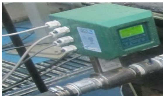
Figure 2: Installing a flowmeter to measure the flow through the radiator
