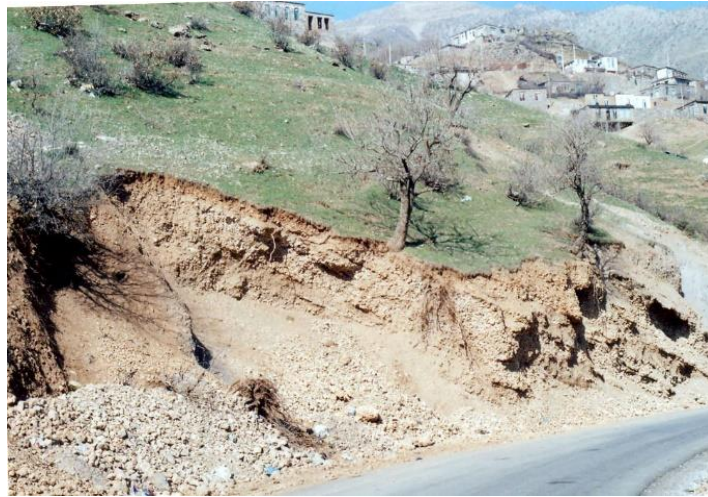
Figure 11. An example of marginal falls located on the sedimentary facies of Garo Formation. Photo of the main road of the basin before Dasheh village - Dideh to the west.
