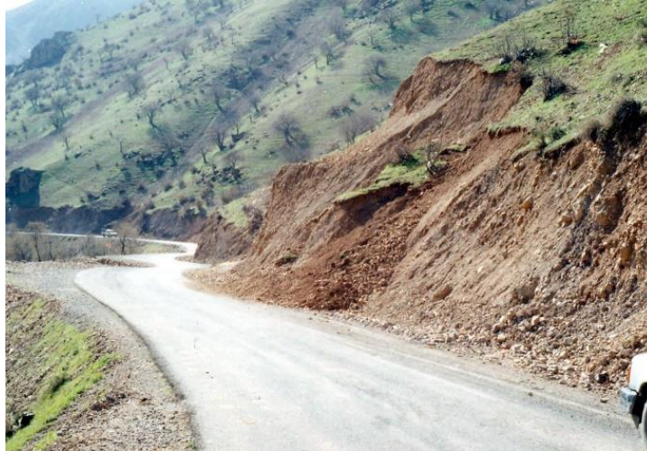
Figure 10. An example of roadside landslides on Jkr rock facies due to road excavation. The fragmented structure of the area shows a high potential for landslides. Photo from Foriab Road to the northwest.
