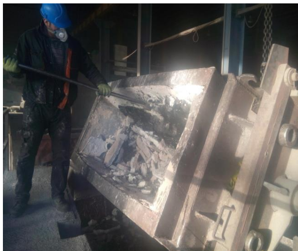
Figure 3) Tundish job demolition workstation after modification
