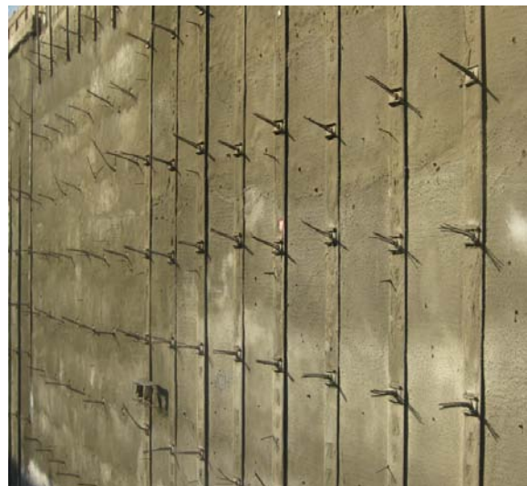
Figure 1. A view of stabilized wall by soil anchorage and steel pile
