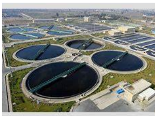
Fig. 1. A view of the Southern Tehran Wastewater Treatment Plant
