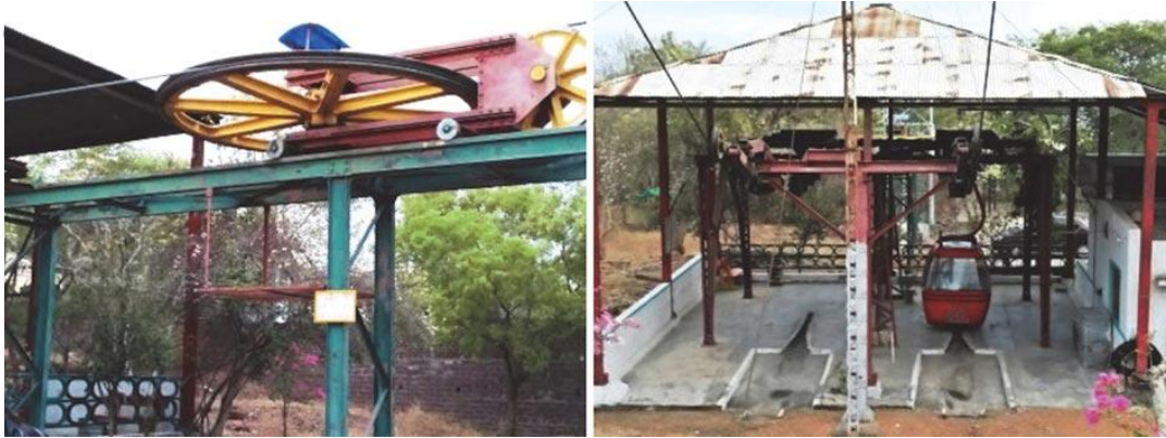
Figure 6- Mechanical System and Passenger Cabin of Bhopal Ropeway at Manuabhan Tekri (photo by authors)
