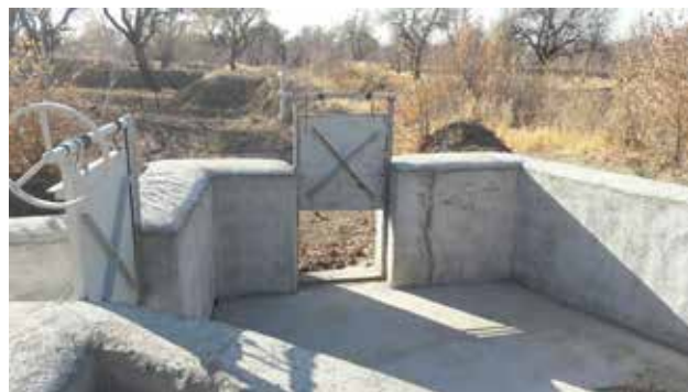
Fig. 3. Water division pool. Photo: Tahereh Salehi, 2017.
