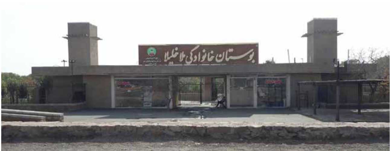
Fig. 6. North entrance of the Garden. Photo: Tahereh Salehi, 2017.
