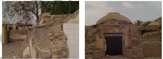
Fig. 8. The comparison of damage to domed mud brick structure and newer built ones (picture taken by author, 2008)
