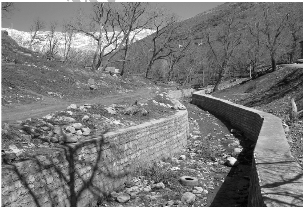
Fig. 2. part of the stream corridor affected by ill-planned developments
