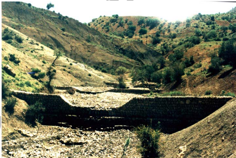
Fig. 1. Buried check dam in the Duroudzan river basin
