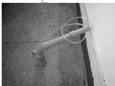
(a) The new type of fluidic sprinkler
