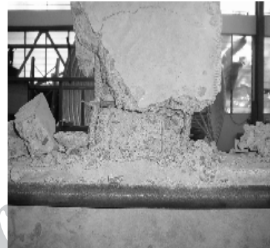
Fig. 6. Observed failure mechanism of specimen CSC1 [12]
