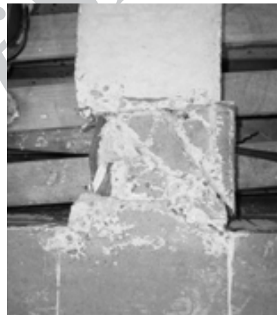
Fig. 11. Observed failure mechanism of specimen RSC1 [12]
