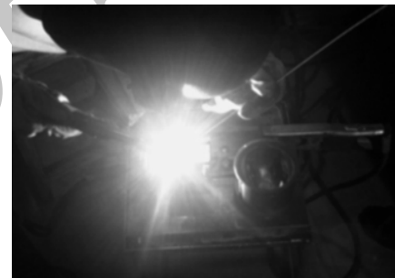
Figure 4. Capping the hole by Argon gas welding
