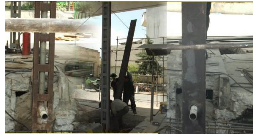
Figure 11. Photo of strengthening construction of a gas station in city of Tehran
