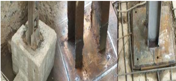
Figure 10. Photo of strengthening construction in a gas station in Tehran
