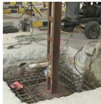
Figure 9. Photo of Foundation Retrofitting
