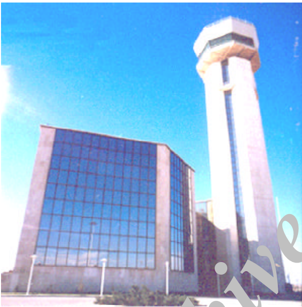
Figure 1. A typical control tower.
