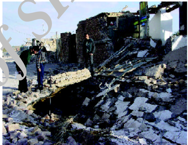
Figure 21. Damage to a building due to collapse of an old hidden Qanat (Baravat).
