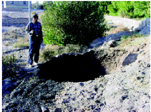
Figure 20. Sinkhole observed close to the main road of Bam to Zahedan near Baravat: same sinkholes induced under the road at the time of earthquake that affected the access of rescue and relief teams to the region.
