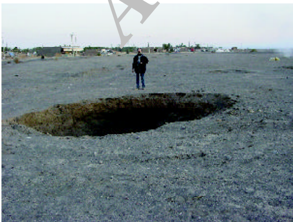
Figure 14. Sinkhole induced due to collapse of a Qanat gallery; west of Baravat
