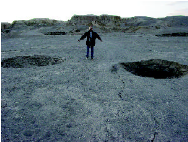
Figure 18. Collapse of shafts and tension crack along the galleries of old Qanats, west of Baravat.
