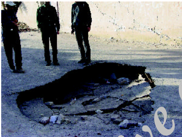
Figure 19. Sinkhole induced due to collapse of an old Qanat on one of the bypasses at Baravat.
