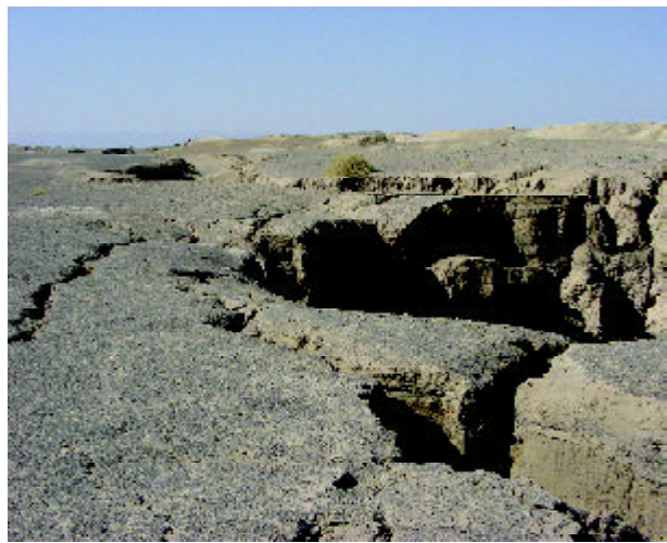
Figure 28. Deep tensional crack and soil blocks fall induced during the earthquake, North of Rahamani village.
