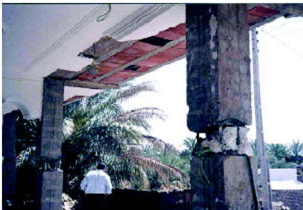
Figure 15. Removing concrete to install stair case.
