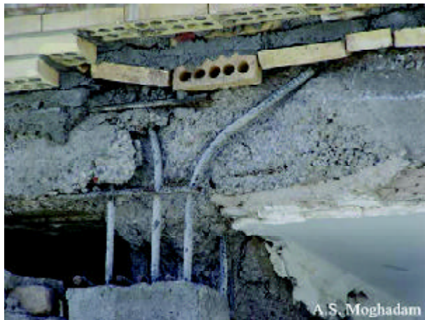
Figure 14. Poor detailing in connection.
