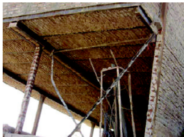
Figure 13. Buckling of bracing and connection damage.
