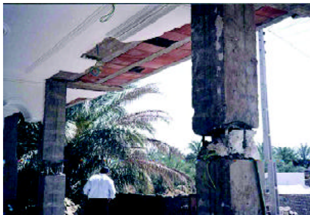
Figure 15. Removing concrete to install stair case.
