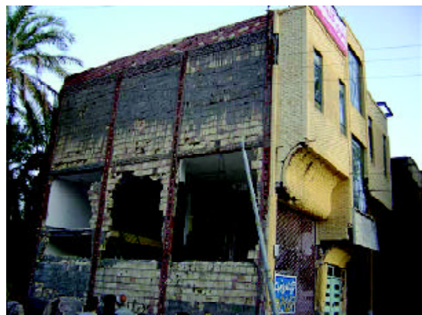
Figure 12. Simple steel frame without bracing.
