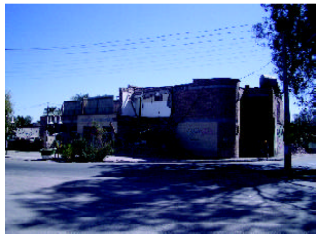
Photo 1. North view of Governor’s building.
