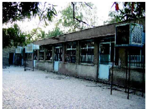
Photo 5. Single-story school building (slight damage).
