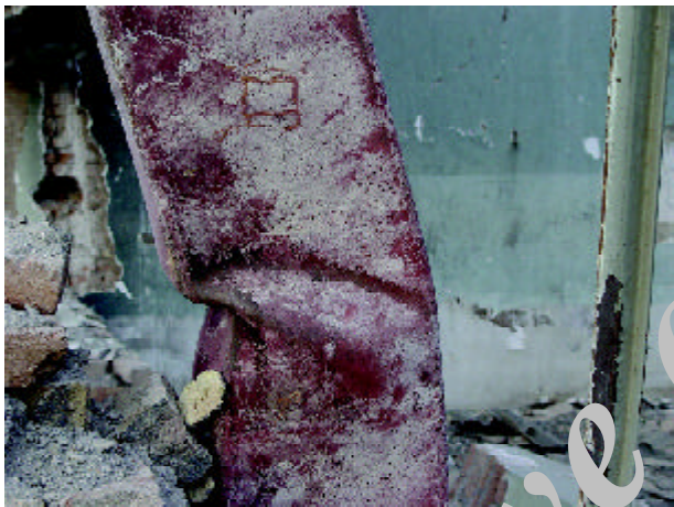
Figure 2. Local buckling of box column.
