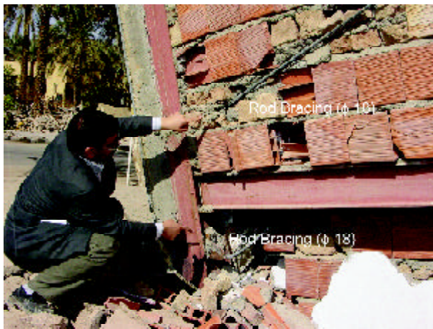
Figure 5. Rod bracings in stories.
