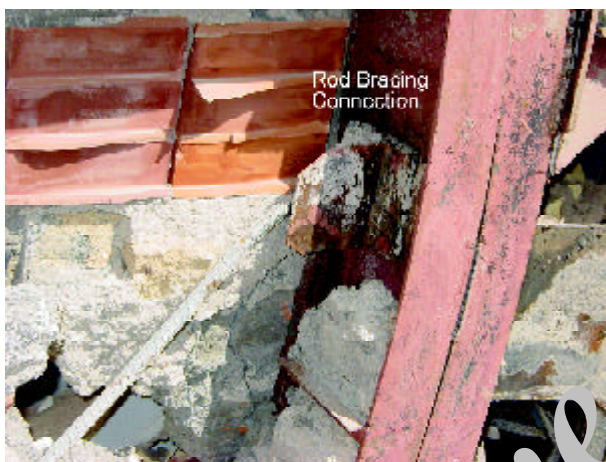
Figure 6. Rod bracing connections.
