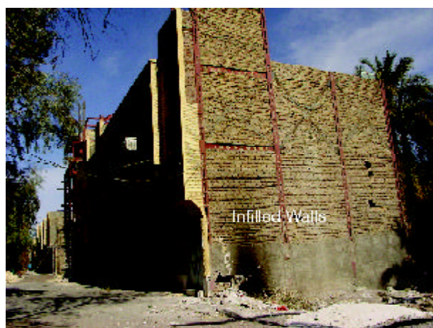
Figure 25. Masonry infill building.
