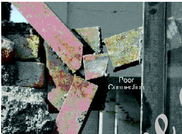
Figure 21. Very poor bracing connections.
