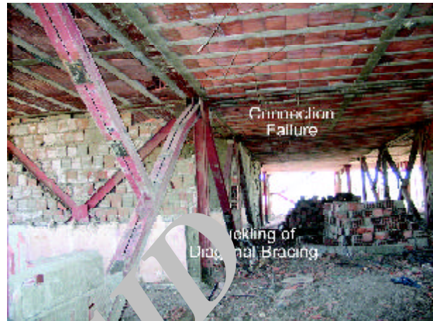
Figure 17. Buckling of diagonal bracings.
