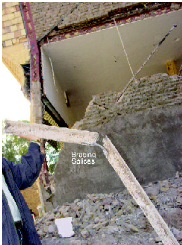
Figure 9. Brace spliced with a rod.
