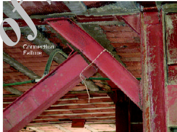
Figure 18. Failure of bracing connections to frame.
