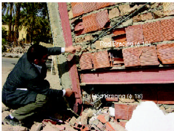
Figure 5. Rod bracings in stories.
