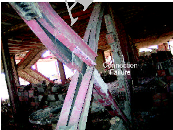
Figure 16. Failure of cross bracing connections.
