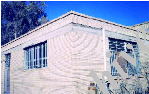
Figure 14. No damage in this code-designed masonry building having ring-beam supported jack arch slab.
