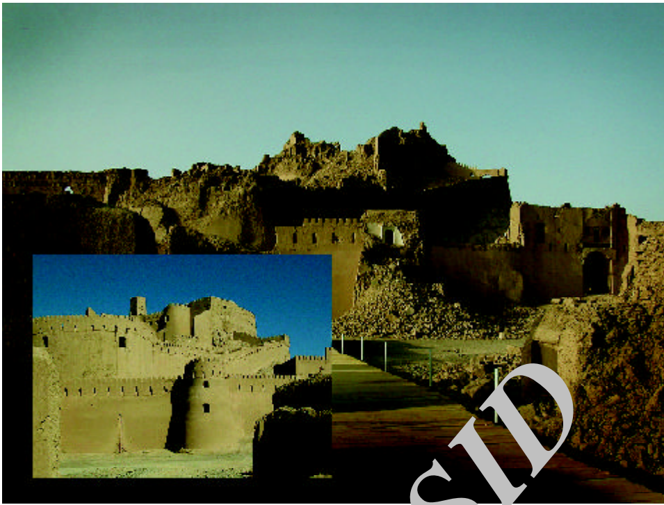
Figure 1. The Arg-e Bam upper citadel before and after the earthquake. Before photo by James Conlon, 2003.
