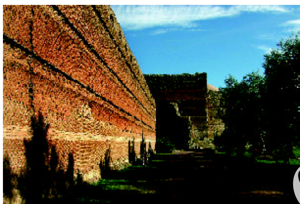
Figure 25. Long Wall, Hadrian's Villa near Rome showing the bands of brick that were laid into a wall constructed with natural cement with a tile facing. The crevices are the result of the later chipping out of the bricks for re-use.
