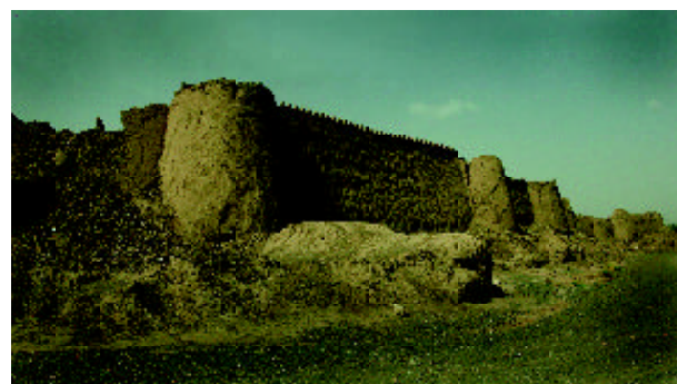
Figure 18. North-facing ramparts that were significantly less damaged in the earthquake than the other city walls. Notice that the crenellations are still intact on this one section, the only section where that was observed to be the case.
