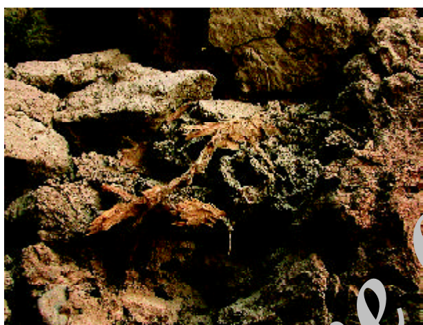
Figure 12. View of section of earthquake-caused collapse showing timber consumed by termites.
