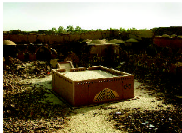
Figures 9 and 10. Before (November 2003) and After (April 2004) of the same view of the Stables courtyard showing the superstructure over the cistern that was recently reconstructed in fired bricks (Before photo by James Conlon, 2003).
