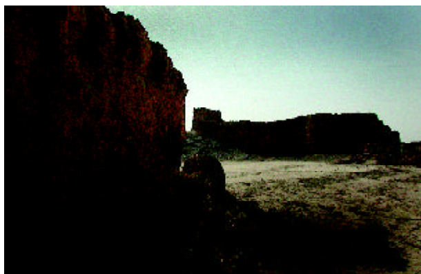
Figure 3. Unrestored ancient earthen structures including the Shahrbast Wall in the distance after the earthquake. These structures were only lightly damaged.
