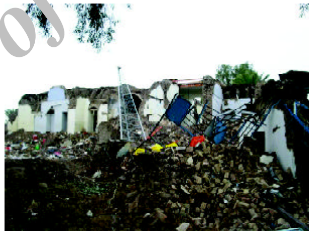
Figures 15. The main telecommunication towers mostly survived the quake. Some communication towers located on roof of the collapsed buildings were also damaged.
