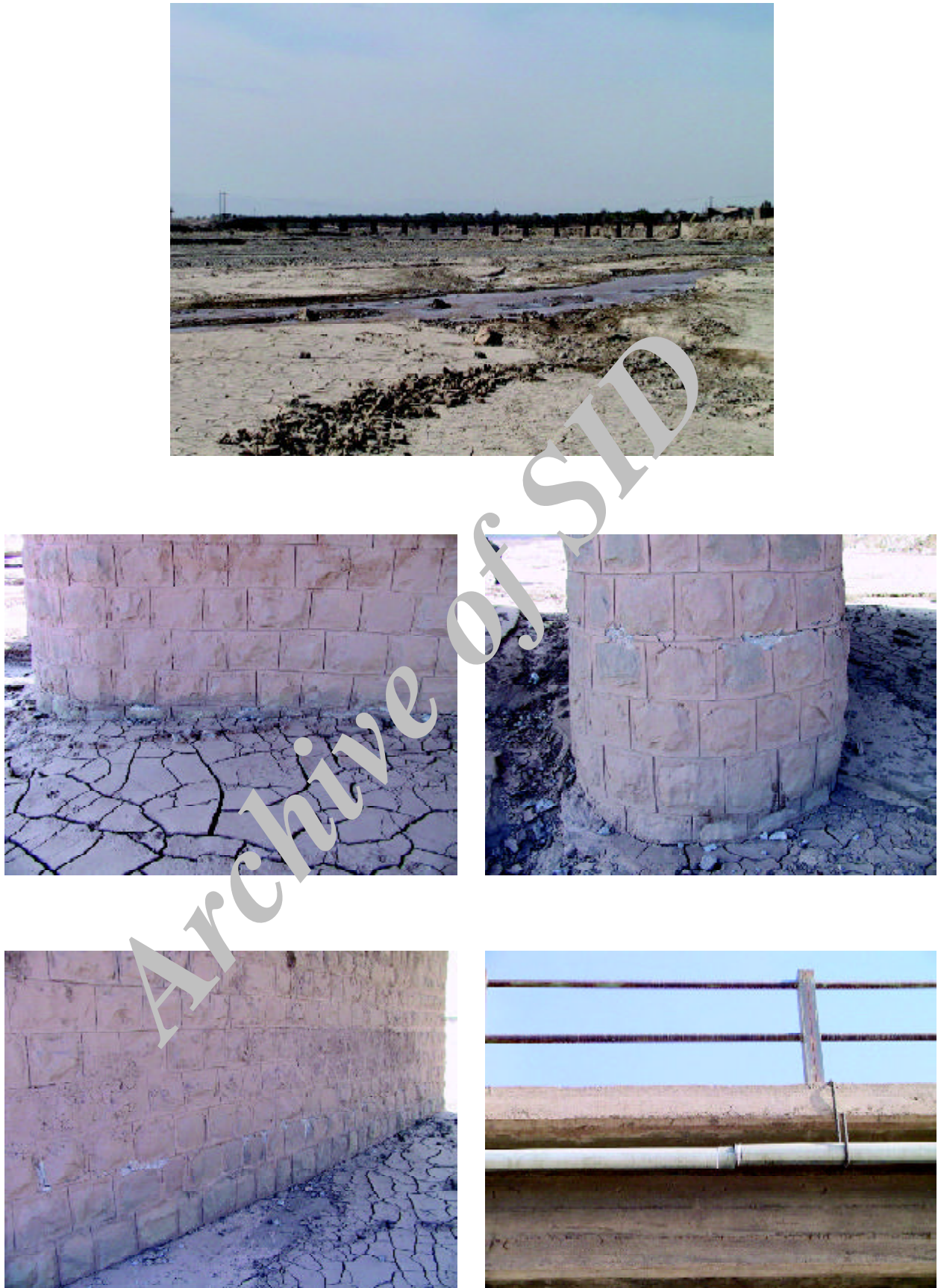
Figure 11. A bridge over the Posht-e-rud performed relatively well. There are signs of vertical movement in the base of the support walls/columns. Damage to pipelines is observed.
