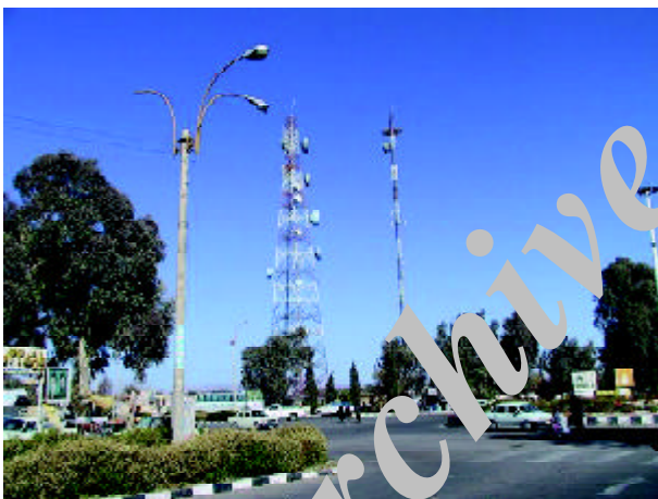
Figures 15. The main telecommunication towers mostly survived the quake. Some communication towers located on roof of the collapsed buildings were also damaged.
