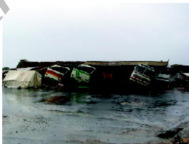
Figure 10. There were minor damage to roads and highways. There were some damage to road embankment and surface cracks cracks in the main highway close to Bam fault scarp. For the most part roads and streets were usable immediately after the quake. The roof of bus terminal building collapsed onto several busses.
