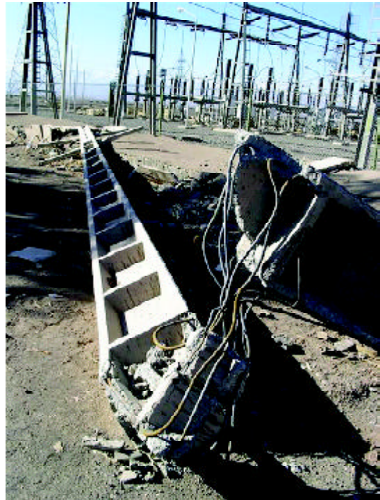
Figure 7. Damage to transmission line towers was not observed. Concrete and wooden poles are used to bring electricity from substations to users. Pole top transformers convert the electricity to 220V. Many distribution poles were damaged. A large number of distribution poles and street light poles were out of plumb after the earthquake.
