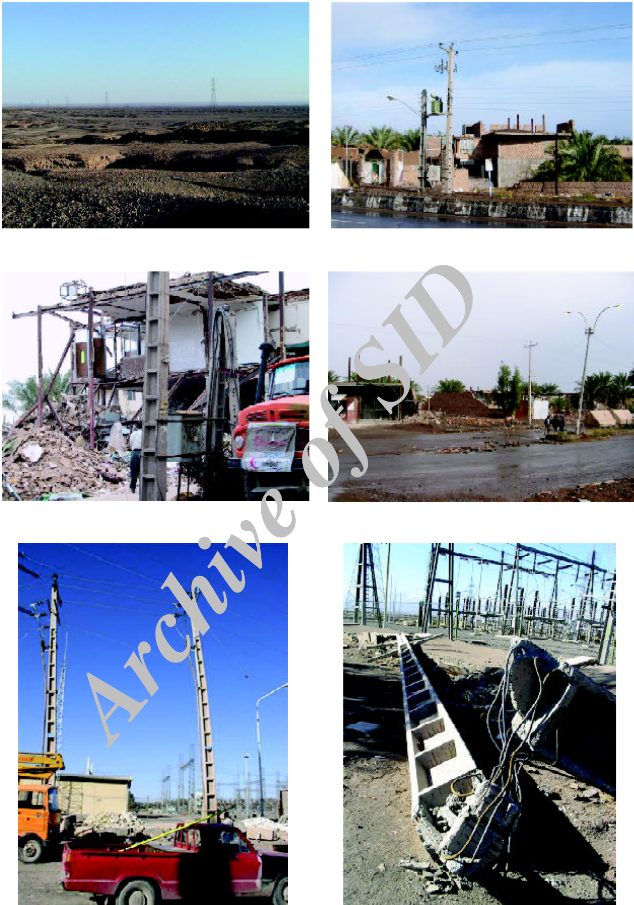
Figure 7. Damage to transmission line towers was not observed. Concrete and wooden poles are used to bring electricity from substations to users. Pole top transformers convert the electricity to 220V. Many distribution poles were damaged. A large number of distribution poles and street light poles were out of plumb after the earthquake.
