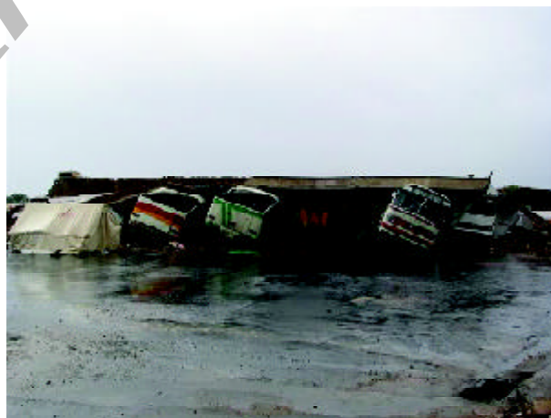
Figure 10. There were minor damage to roads and highways. There were some damage to road embankment and surface cracks cracks in the main highway close to Bam fault scarp. For the most part roads and streets were usable immediately after the quake. The roof of bus terminal building collapsed onto several busses.
