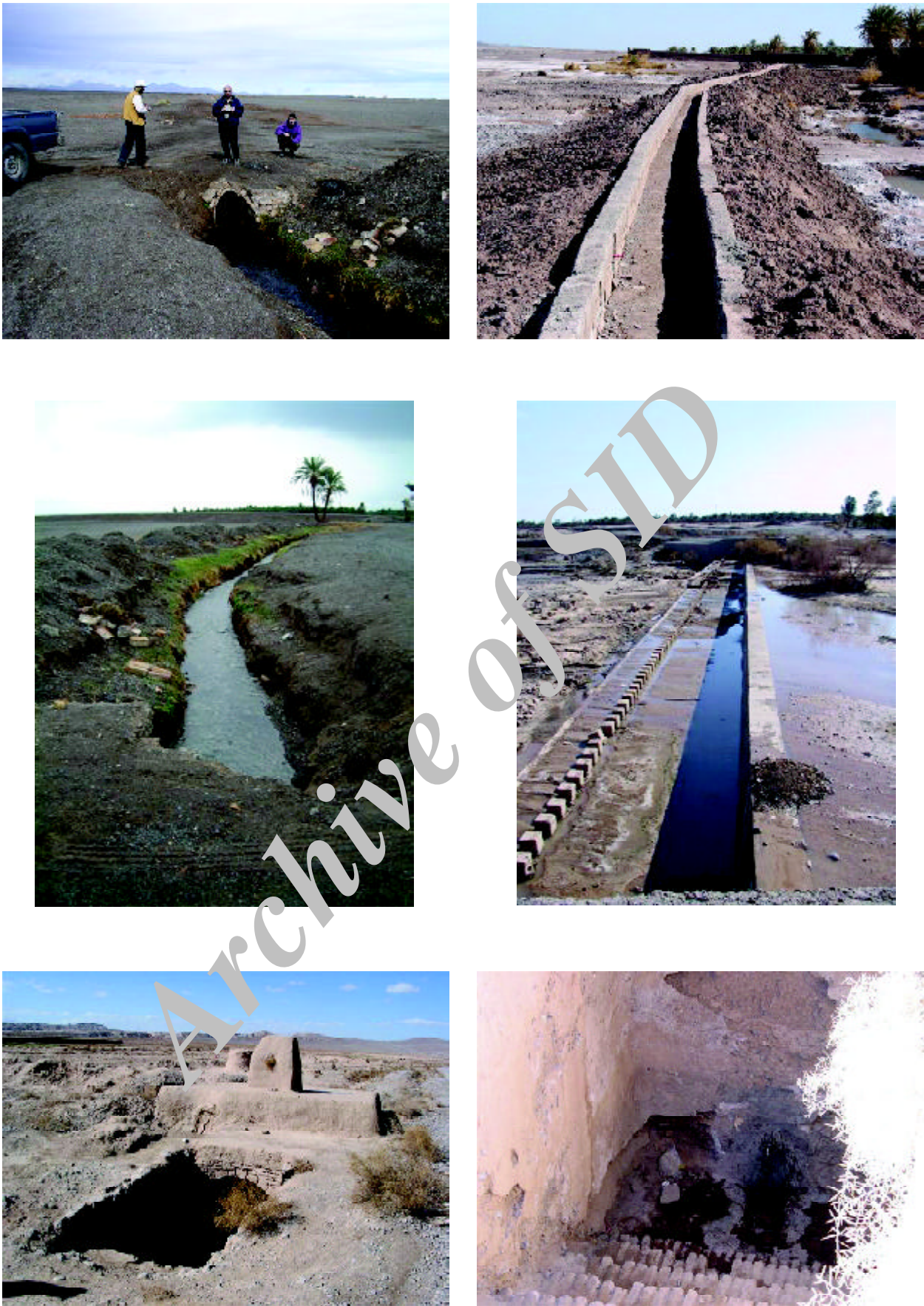
Figure 5. Once the qanat chain arrives at its destination, the underground tunnel reaches the ground surface (top and middle left pictures). From there the water is distributed via man-made channels and brought to farms and date palm gardens. Damage to the channels is noted in the middle and lower right pictures. The qanat water sometime is stored in traditional underground reservoirs (bottom two pictures).
