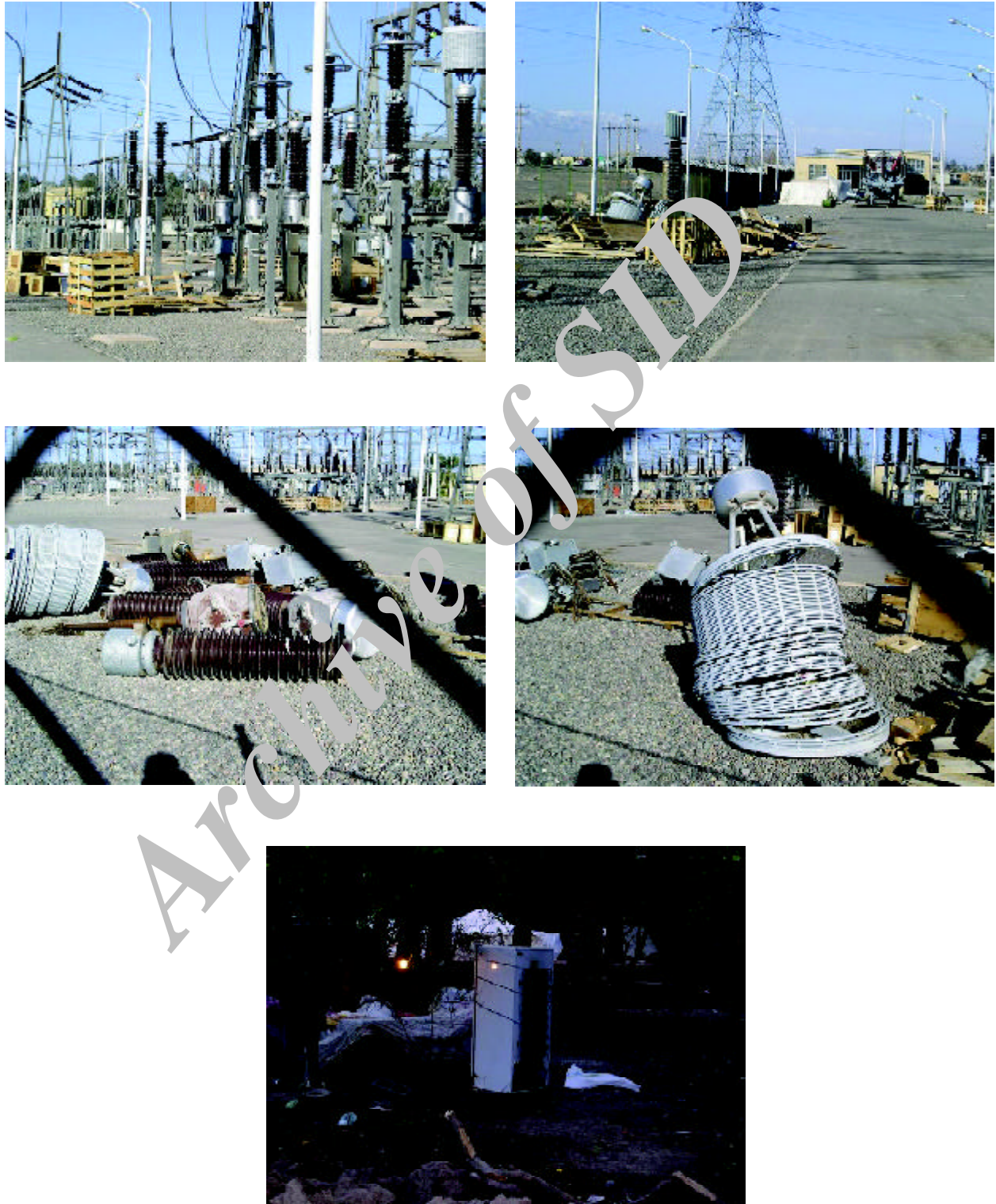
Figure 9. Damage to various electric equipments in the 230kV substation is observed in the above pictures. At the time of our visit (one month after earthquake) the electricity was available throughout the city, even though most of the users' buildings had been severely damaged to use the electricity.
