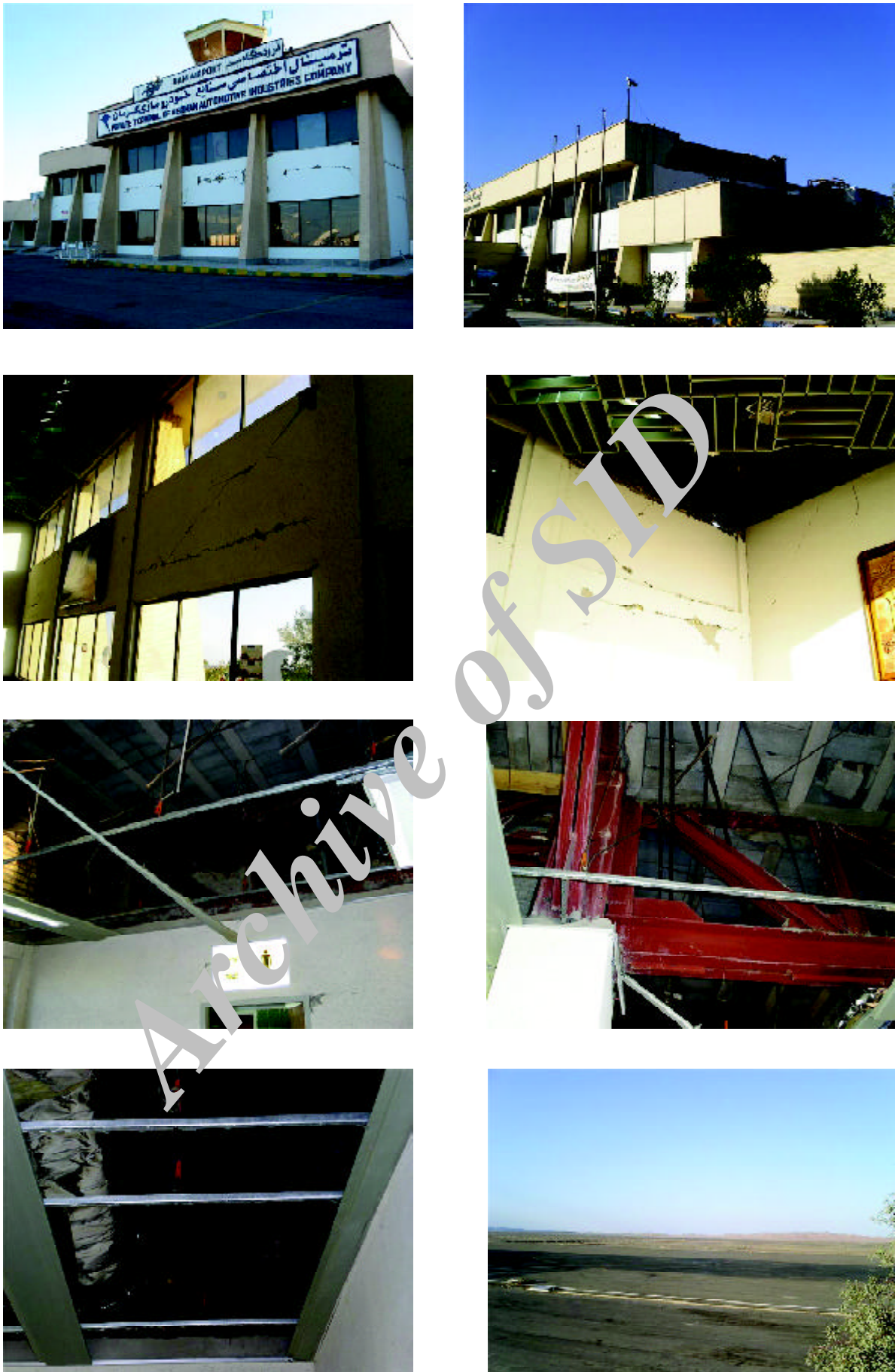
Figure 12. The engineered steel frame terminal building at Bam airport was moderately damaged. The masonry infill walls were damaged. The false ceilings were severely damaged. The airport runway had little damage.
