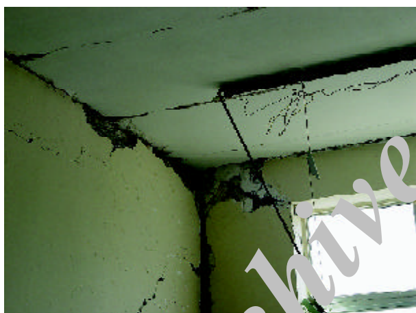
Figure 47. The failed light fixtures in the office building of the city electric power substation (Photo by M. Hosseini).
