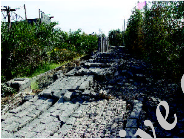
Figure 7. Topped concrete block (partially brick) wall (Photo by M. Hosseini).
