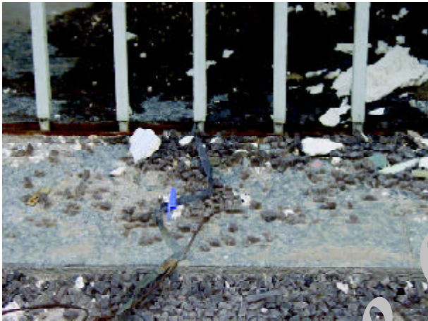
Figure 33. Splashed Parts of the broken thick glass of Bank Refah Karekaran building (Photo by M. Hosseini).
