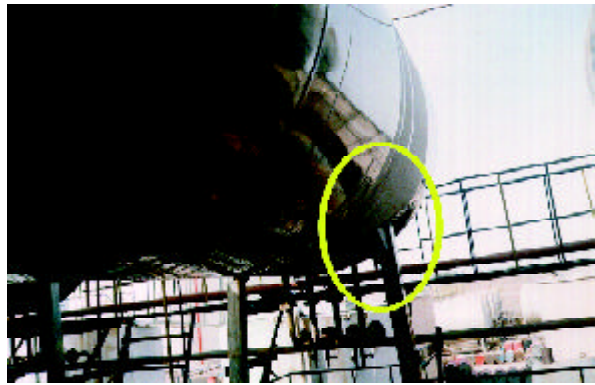
Figure 22. Punching of tank shell [1].
