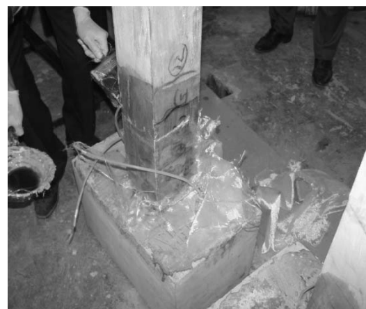
Fig.9 Installation of prefabricated composit sheets
