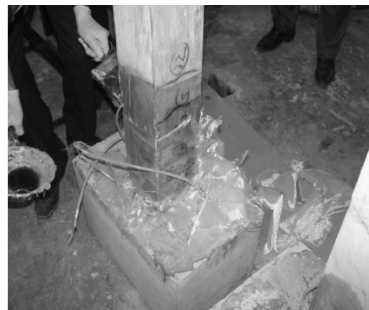
Fig.9 Installation of prefabricated composit sheets
