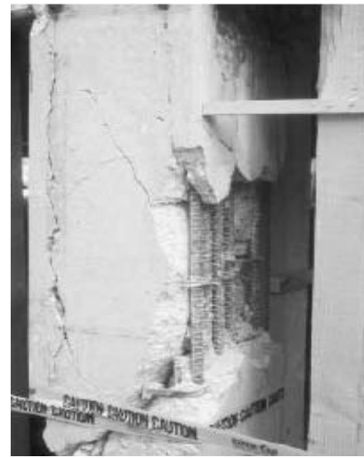
Fig.2 Failure of lap splice due to insufficient splice length and widely spaced ties with 90° hooks (Northridge-1994)
