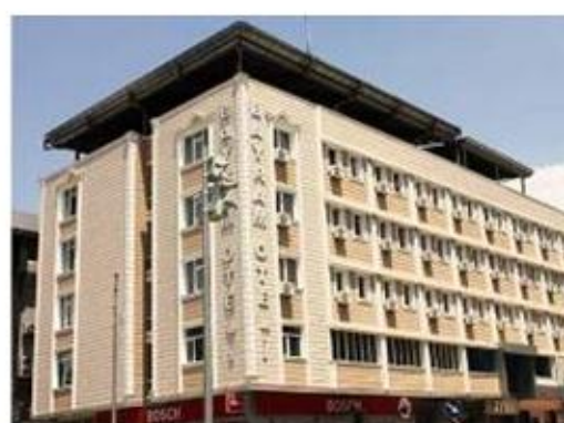
Fig. 2: Hotel Bayram of Van, before (down) and after (up) of its collapse in the aftershock of 9 November 2011, M5.6 (3, 4)
