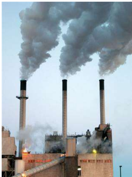
Fig. 2-b: Emissions from coal-fired power plants include sulfur dioxide, mercury, nitrogen oxides and carbon dioxide, Phillip J. Redman / U.S. Geological Survey (19)
