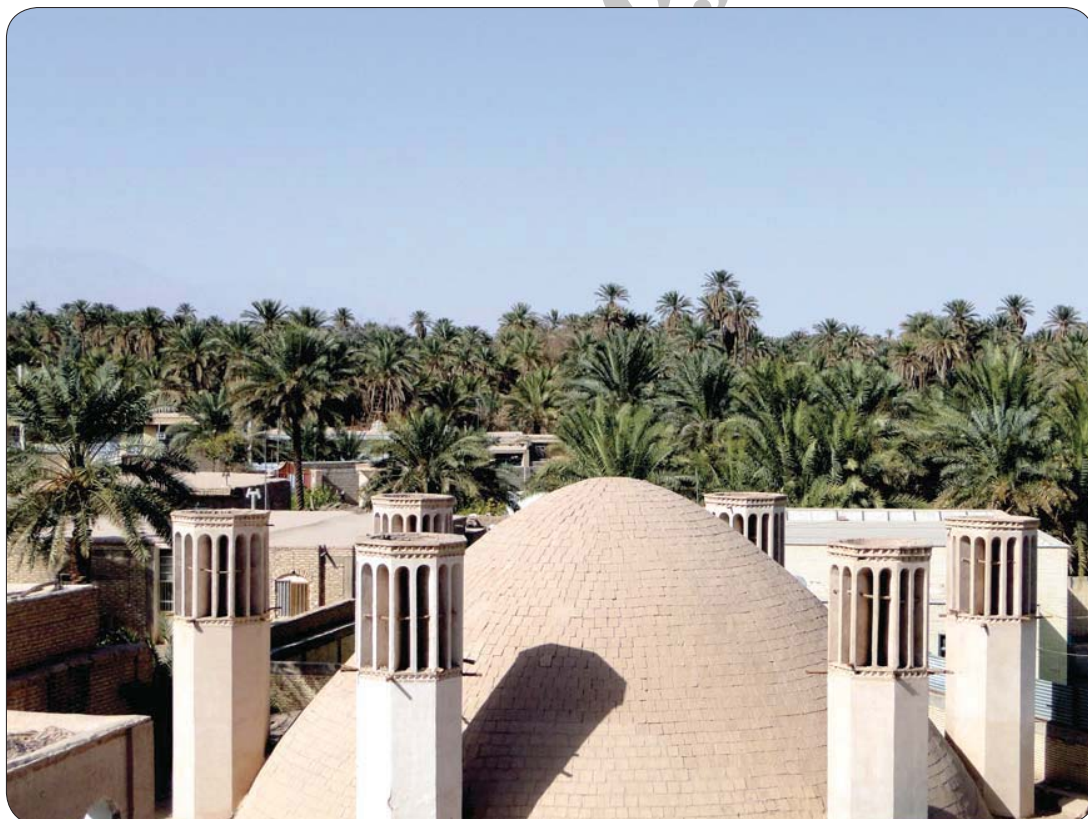
The dome of a traditional drinking water reservoir (Ab anbar) with six windcatchers, Shahdad, 96 Km from Kerman, Kerman Province, Iran (Photo by S. Borzabadi Msc, 2012).
