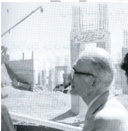
Figure 8. Two photos of the construction of the Kerman University in 1970s. 6
