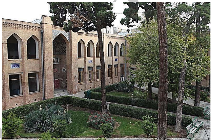
Figure 5. A recent view of the Dar al-Fonun School, founded in 1851. (Photo by: Mr. Jamshid Rabeei). 6
